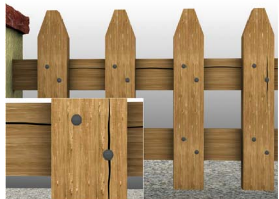
Fig. 19. Wood gate with cracks created by weathering of nails
